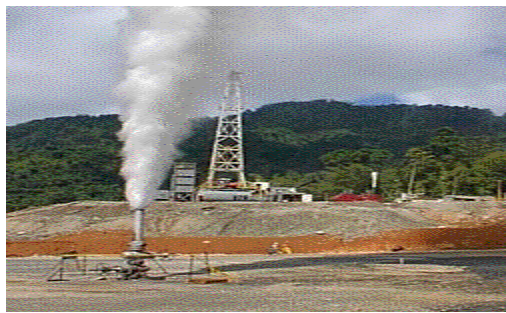
Geothermal wells are drilled to help reduce pit temperature
